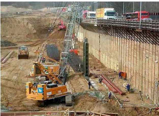
PICTURES ABOVE AND RIGHT ARE EXAMPLES OF CUT & COVER TUNNEL WORKS
