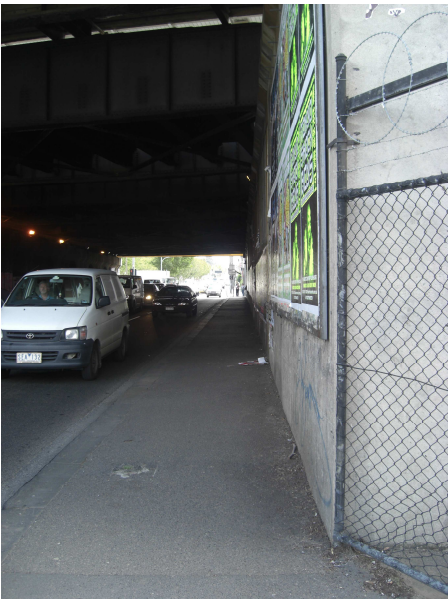
General tunnel conditions Conditions within the tunnel are extremely poor. Footpath width appears to be insufficient. Dim lighting and graffiti / posters contribute to the poor conditions.
