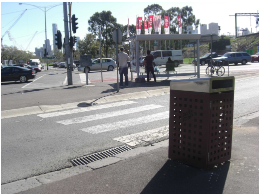
Swan Street / Punt Road intersection No tactile pavement is provided. Vehicles were observed to queue across zebra crossing. Bus stop is located within traffic island.
