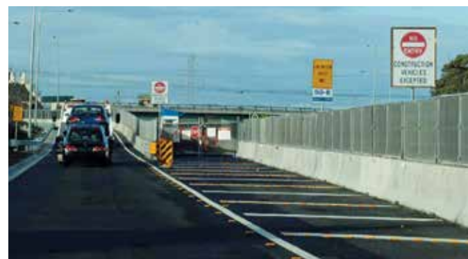
Figure 6-28: Access to the works within the operating freeway could be either through the section of completed tunnel from a work site, or by entry directly off the freeway lanes
