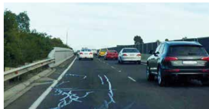
Figure 6-27: An example of traffic lanes being diverted onto the road shoulder, with a barrier separating construction from traffic
