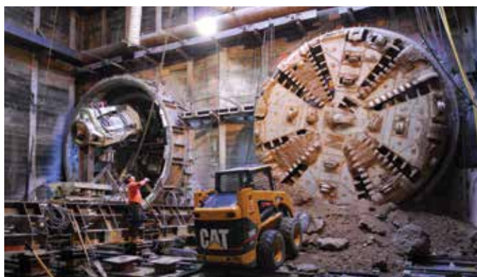
Figure 6-26: A Tunnel Boring Machine (TBM) similar to that which could be used to construct a Rapid Transit Option underneath the CBD
